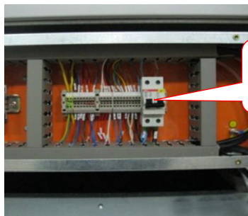
Prime power connections to WPU
