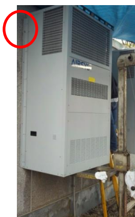
Figure 8: Verify the Unit is Level
