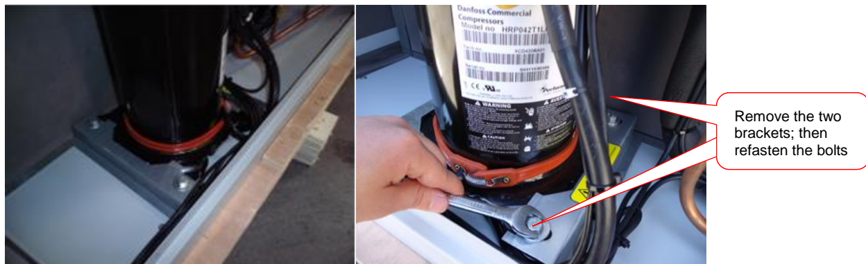
Figure 12: Remove Compressor Brackets
